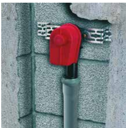
Wandmontage: Wasmachine-sifon
